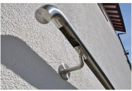
Carry out adjustments to the hand rail, such as cutting or welding, directly on-site.
