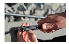
Loop the LED light bar through the handrail supports, introduce into the groove and click into the adapters
